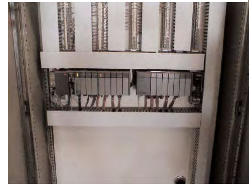
DC-Powered PLC and I/O with Four Motor Drives
