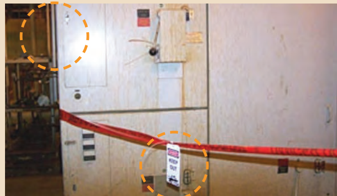
Figure 2: Highlighted on the top left is the racking handle for R1 starter, and bottom right is the racking handle for Q101 ("M" starter).
